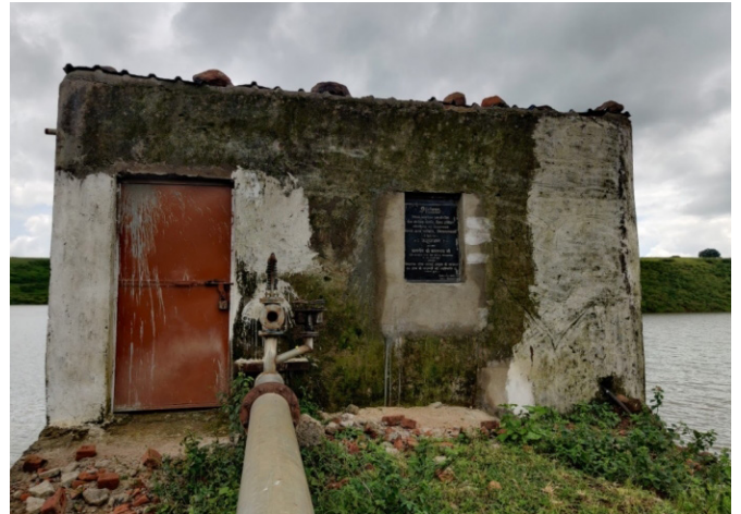
Lift irrigation pump in Jamai
